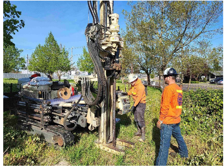
AEC setting up 7822 DT drill rig to complete boring
