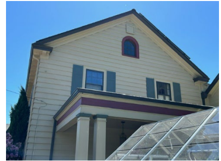
Figure 7 Upstairs main house north facing (2 windows)
