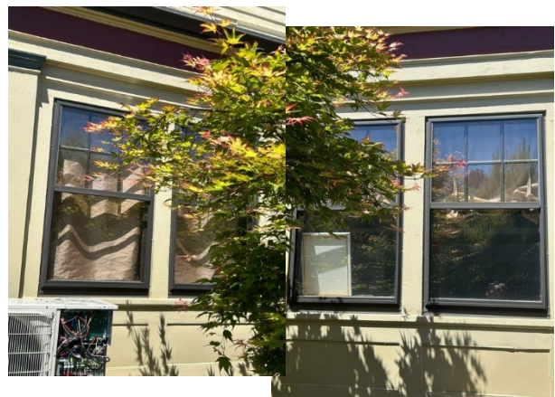
Figure 4 Sunroom 9th Ave facing (4 windows)
