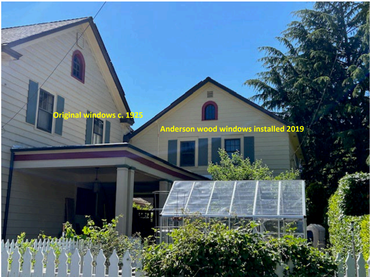
Figure 8 Original windows and Anderson 400 series wood windows on 2019 addition
