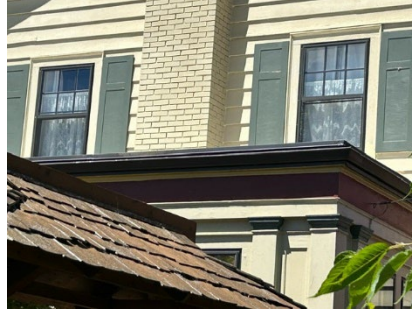
Figure 6 Upstairs main house 9th Ave facing (2 windows)
