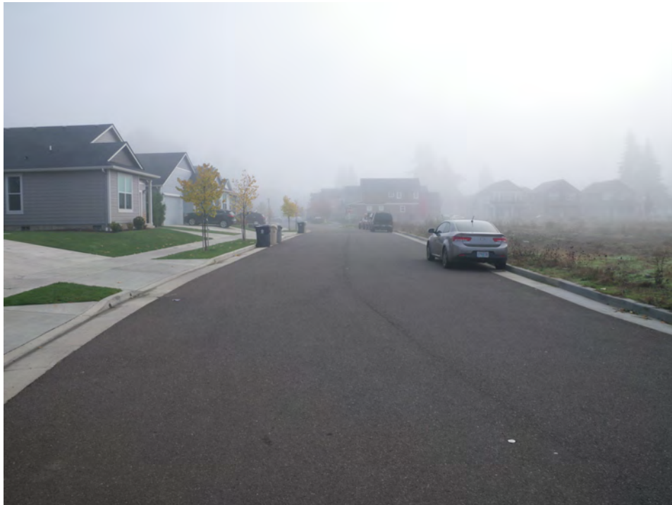
Front Avenue, looking east. Subject is at right
