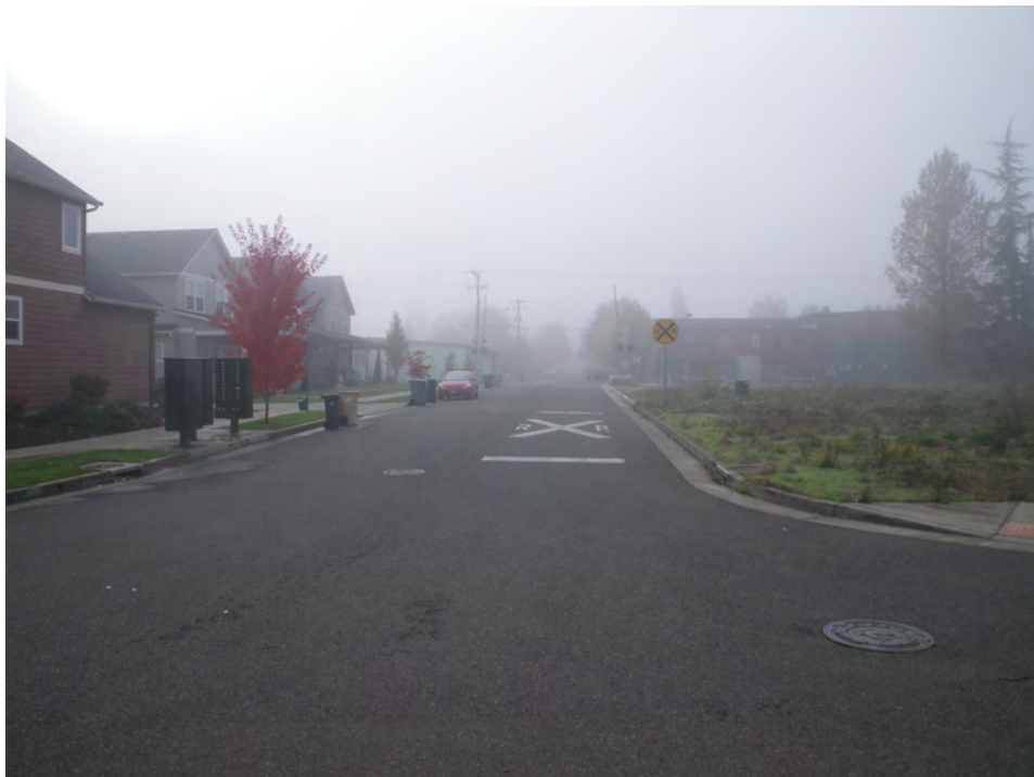
Hill Street, looking south. Subject is at right
