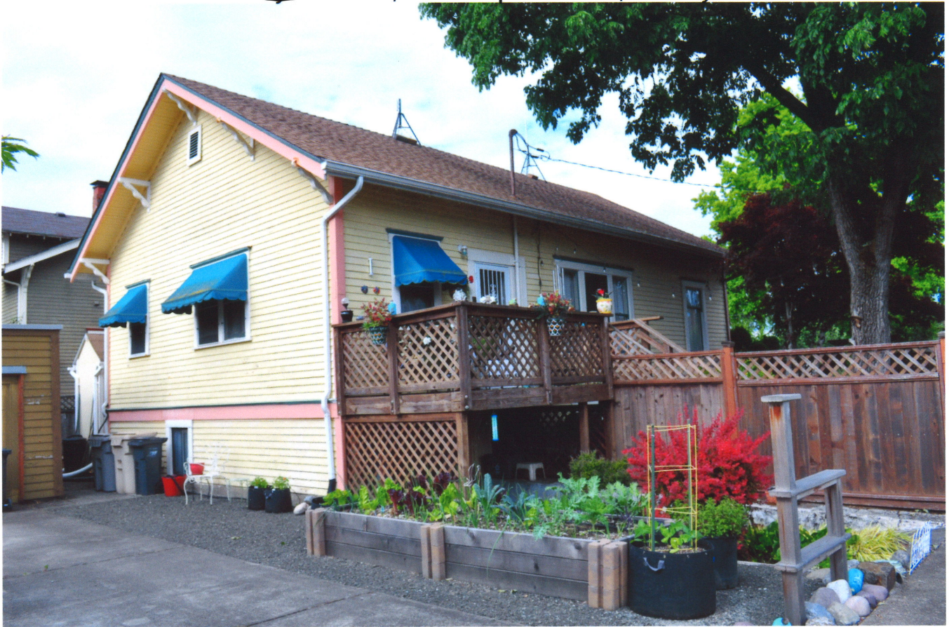
West and South Walls Overview (deck is off south wall)
