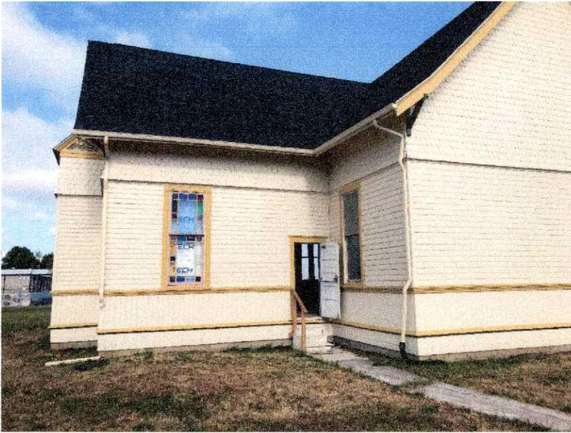
Southeast Façade Showing Subject Window
