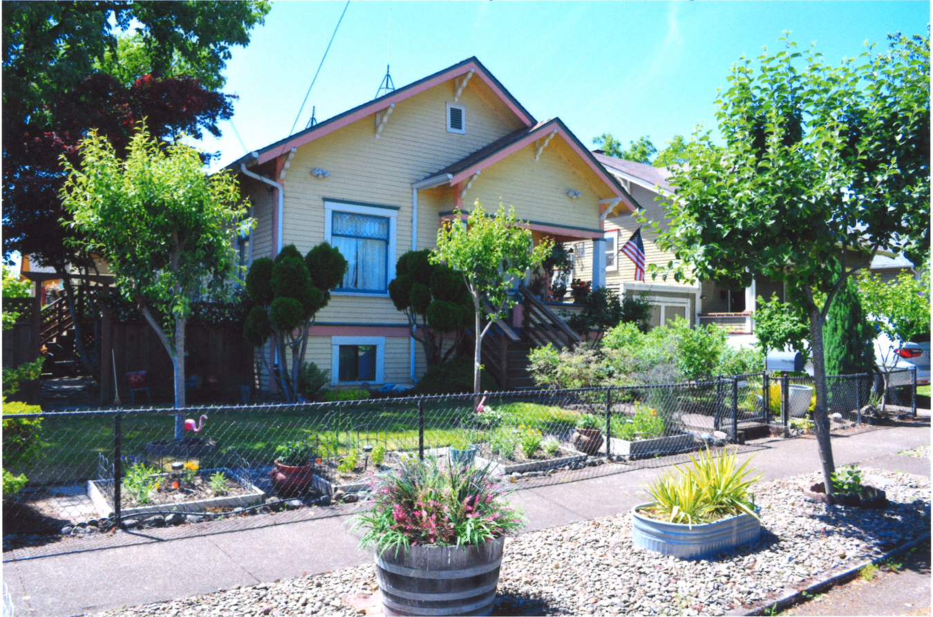
North Front Entrance and South Wall Overview
