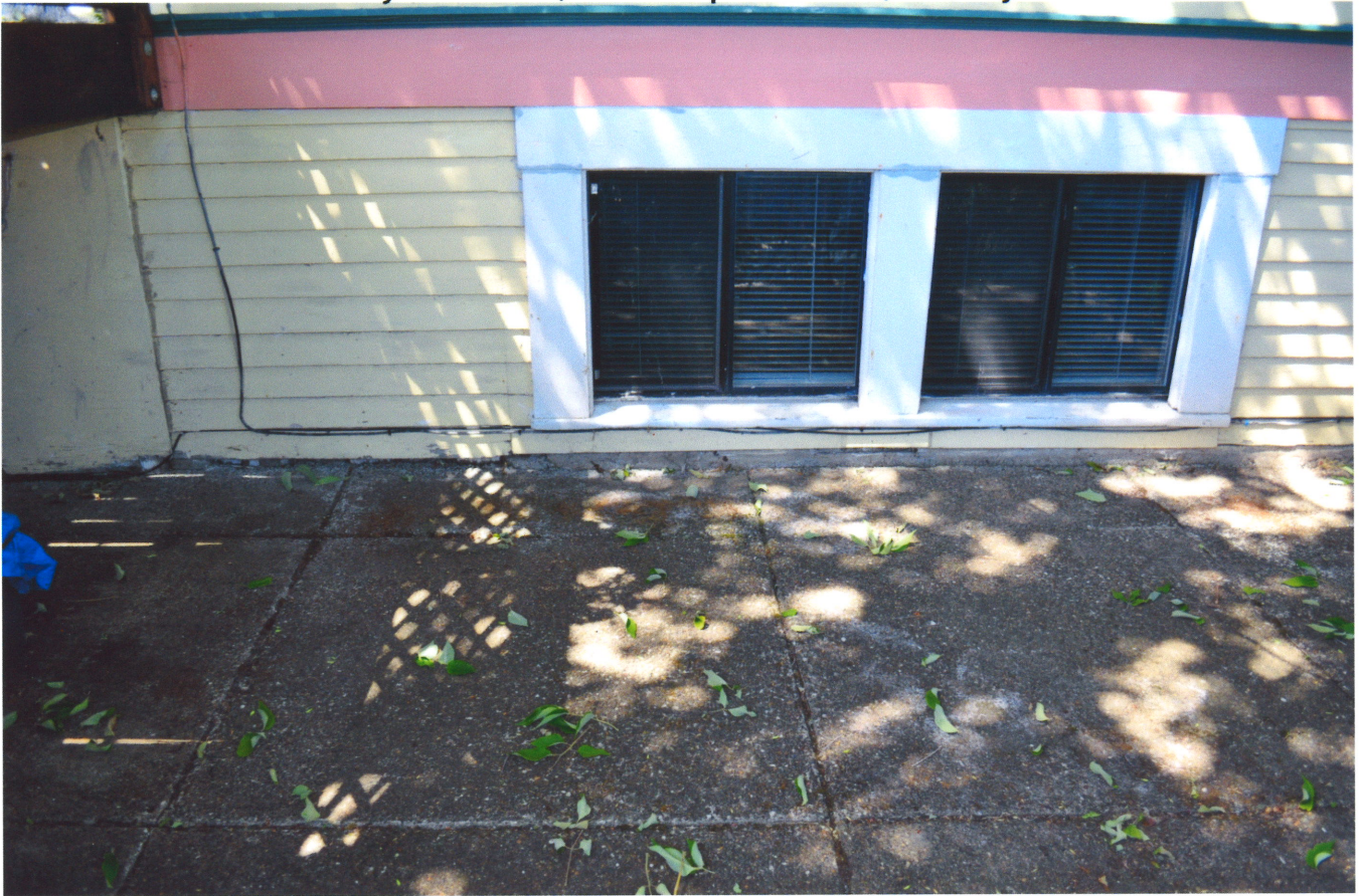
South basement wall where French drain will be installed
