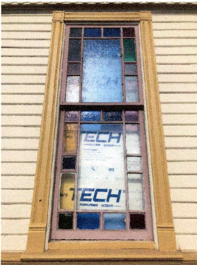
Subject Window – Exterior View
