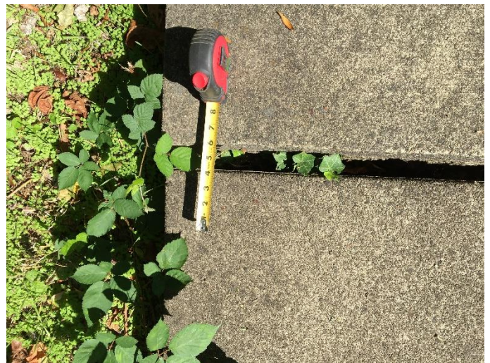
Between Ellsworth & Lyon, slab panel lateral offset
