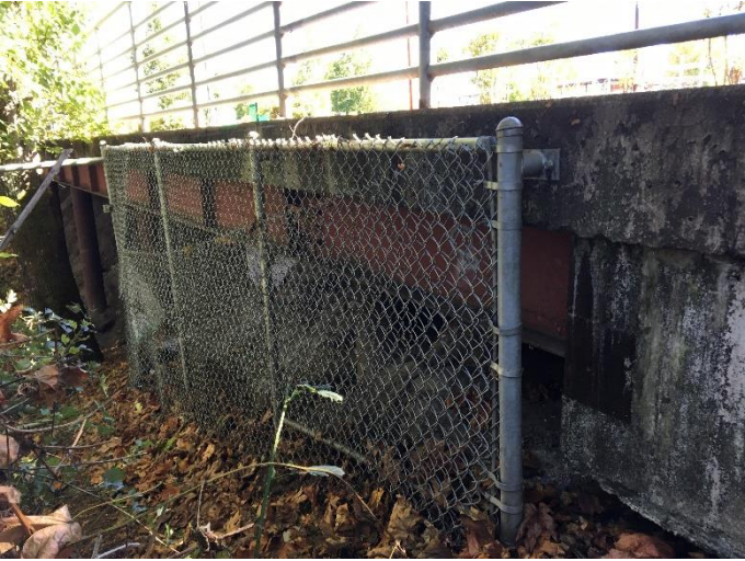
Between Montgomery & Railroad, trail transition to pile-support
