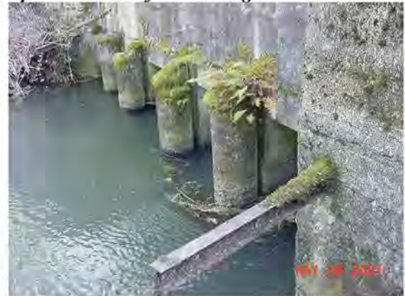
Photograph 7-7: Abandoned Gate Guides on Upstream Side of Old Headgate
