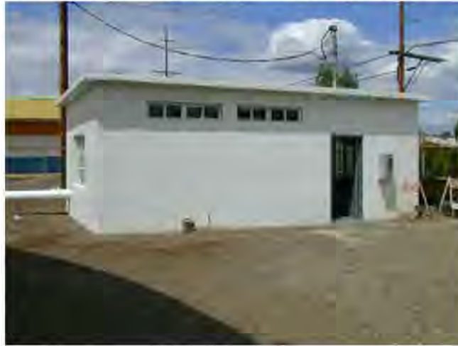
Photograph 3-4: Queen Avenue Pump Station
