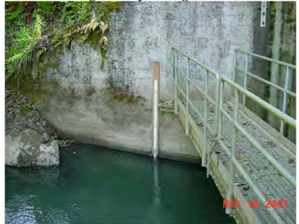
Photograph 7-4: View of Upstream Staff Gage on South Wing Wall of Headgate
