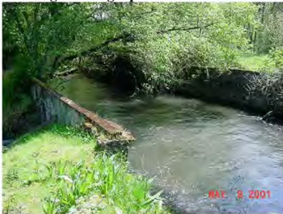
Photograph 7-14: Canal at Cox Creek Crossing Looking Upstream
