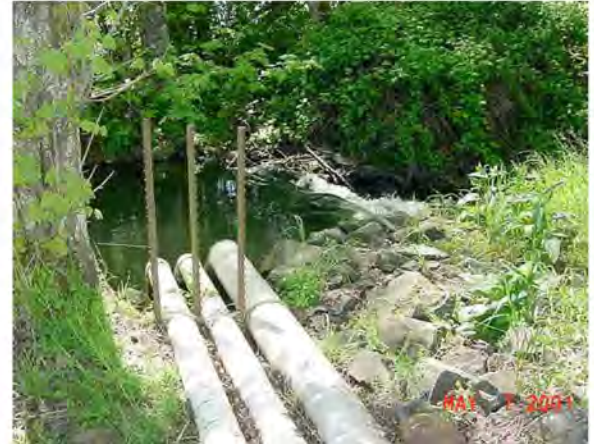
Photograph 7-17: Irrigation Siphon Pipes
