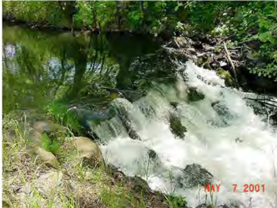
Photograph 7-16: Rock Check Dam in Channel
