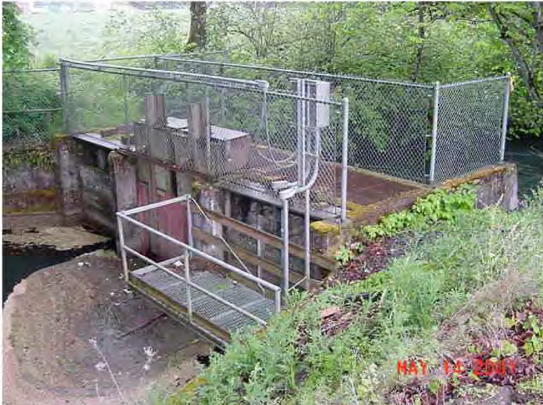
Photograph 7-13: Upstream Side of Albany Gates
