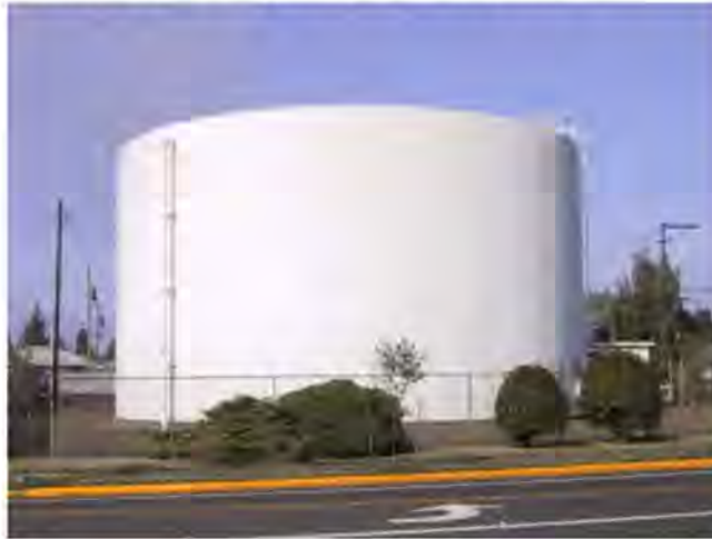
Photograph 3-9: Queen Avenue Reservoir
