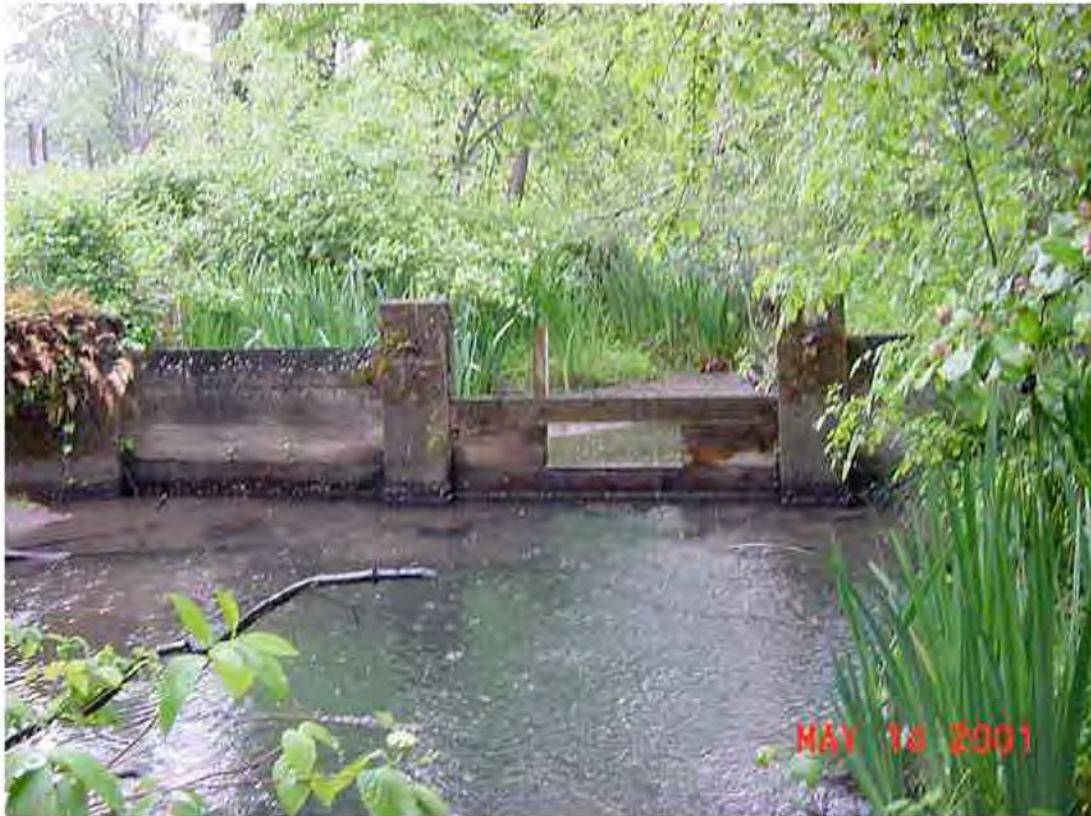
Photograph 7-12: Overflow Weir to CZ Tailrace (Hospital Slough)
