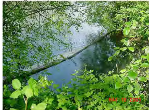
Photograph 7-2: Canal Point of Diversion and Logboom (RM 20.9, Canal Sta 0+00)
