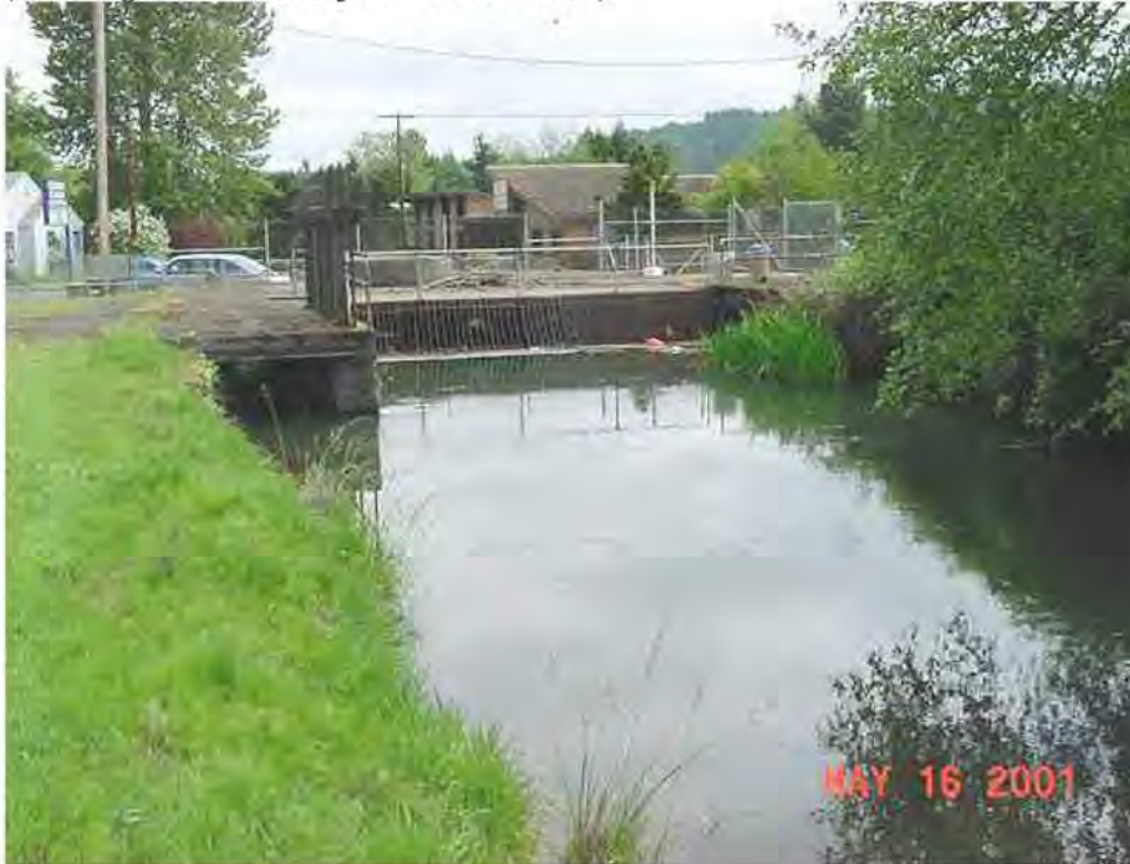
Photograph 7-8: Overview of intake at Lebanon WTP (Looking Downstream from WTP Intake)
