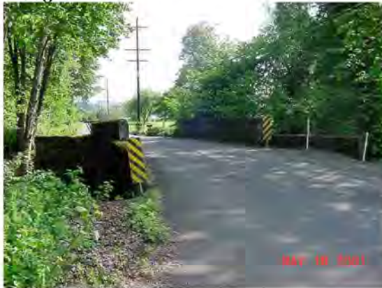
Photograph 7-6: Top View of the Old Headgate
