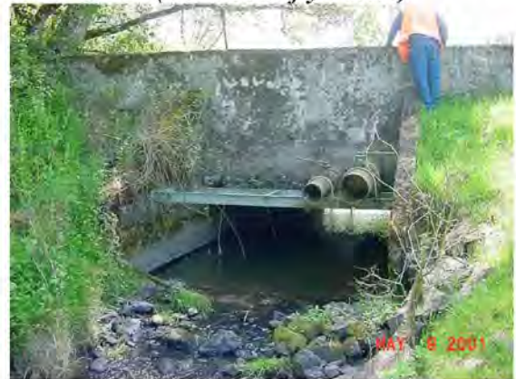
Photograph 7-15: Cox Creek Culvert Passing Under Canal (Note Butterfly Valves)
