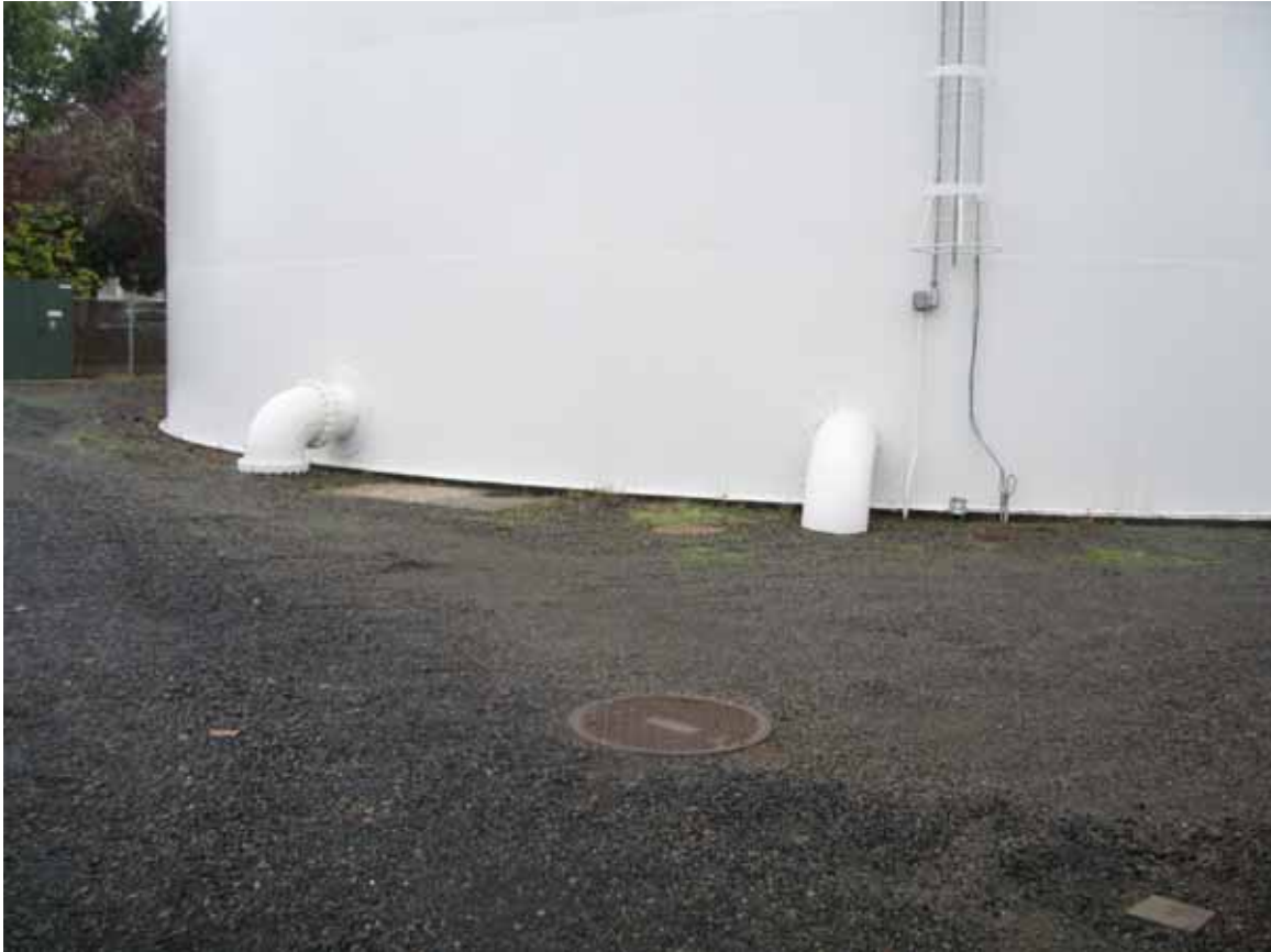
Figure 5-18. Two of three Inlet-Outlet Pipes for Maple Reservoir
