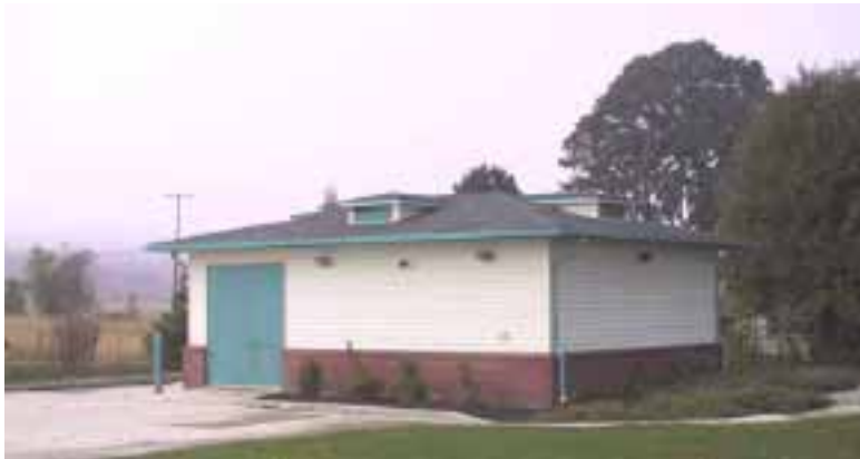
Figure 2-9. Gibson Hill Pump Station
