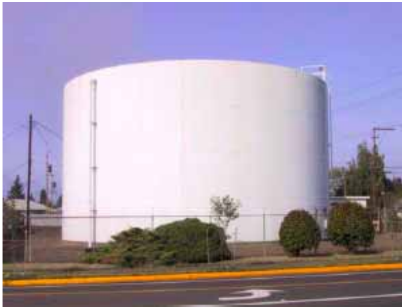
Figure 2-12. Queen Avenue Tank
