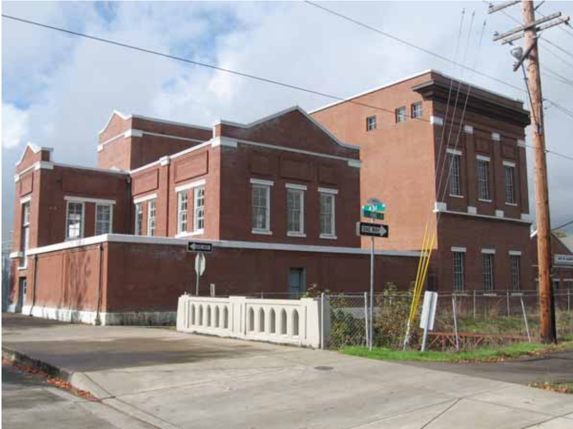
Figure 5-6. Old Filter Building (Left Side) and Soda Ash Building (Right Side)
