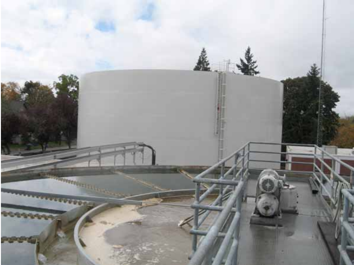
Figure 5-17. Maple Reservoir (Background), Accelerator 2 (Foreground)
