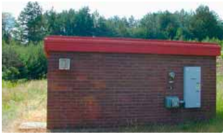
Figure 2-8. North Albany Pump Station
