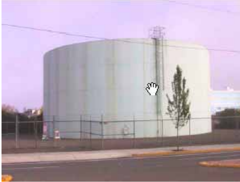
Figure 2-13. 34 th Avenue Tank
