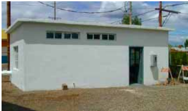
Figure 2-7. Queen Avenue Pump Station
