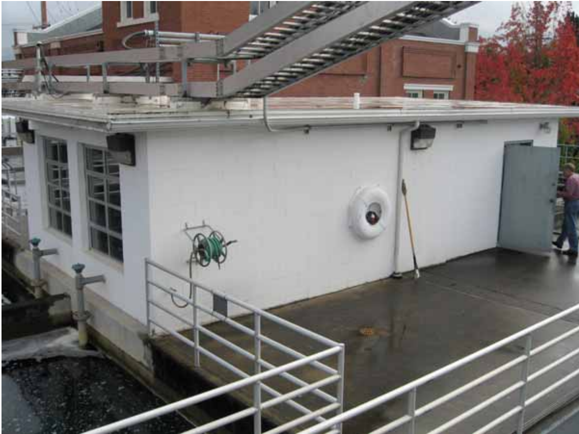
Figure 5-9. CMU Building – Large Filters
