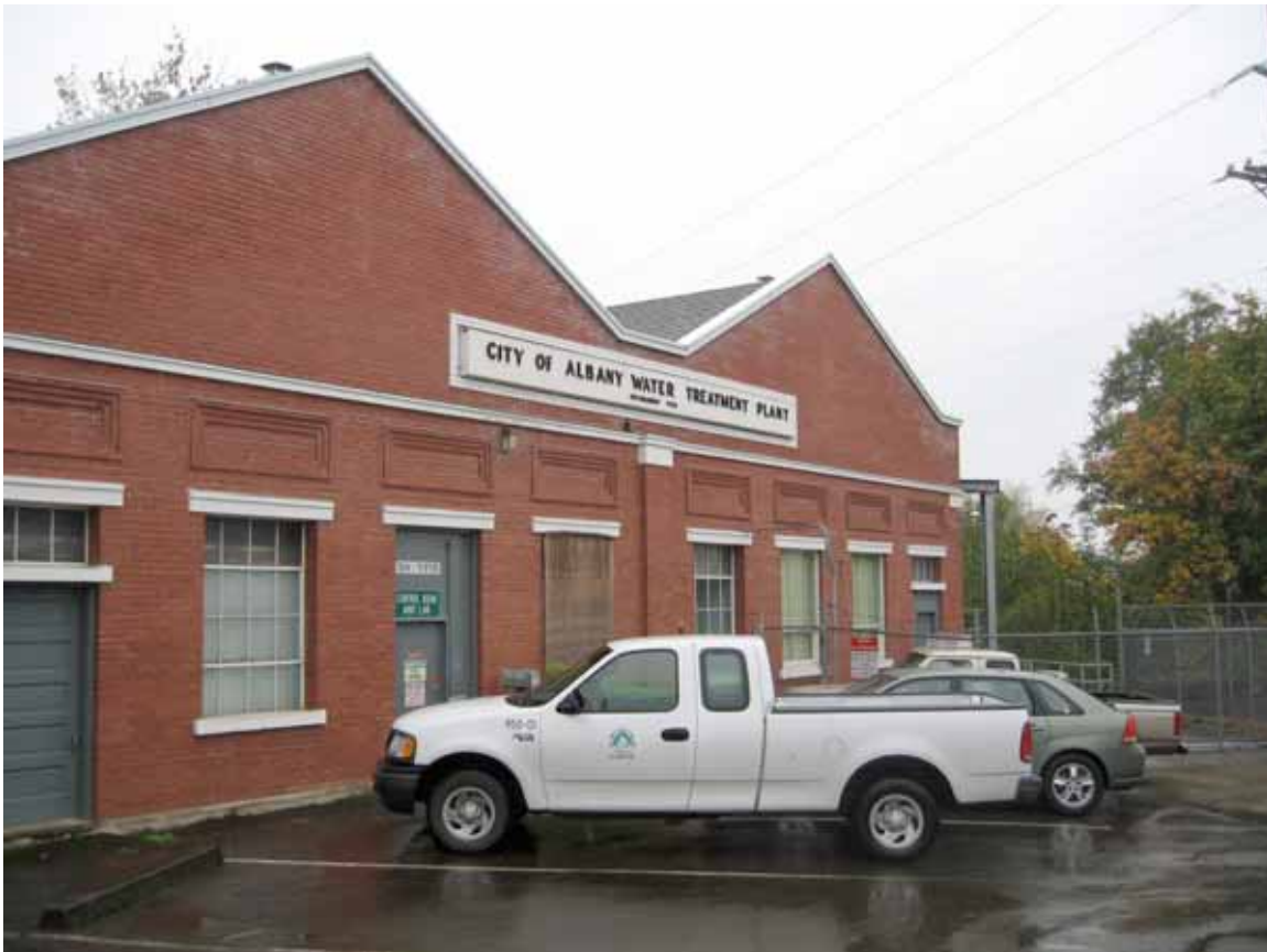
Figure 5-1. Control Building, East Elevation
