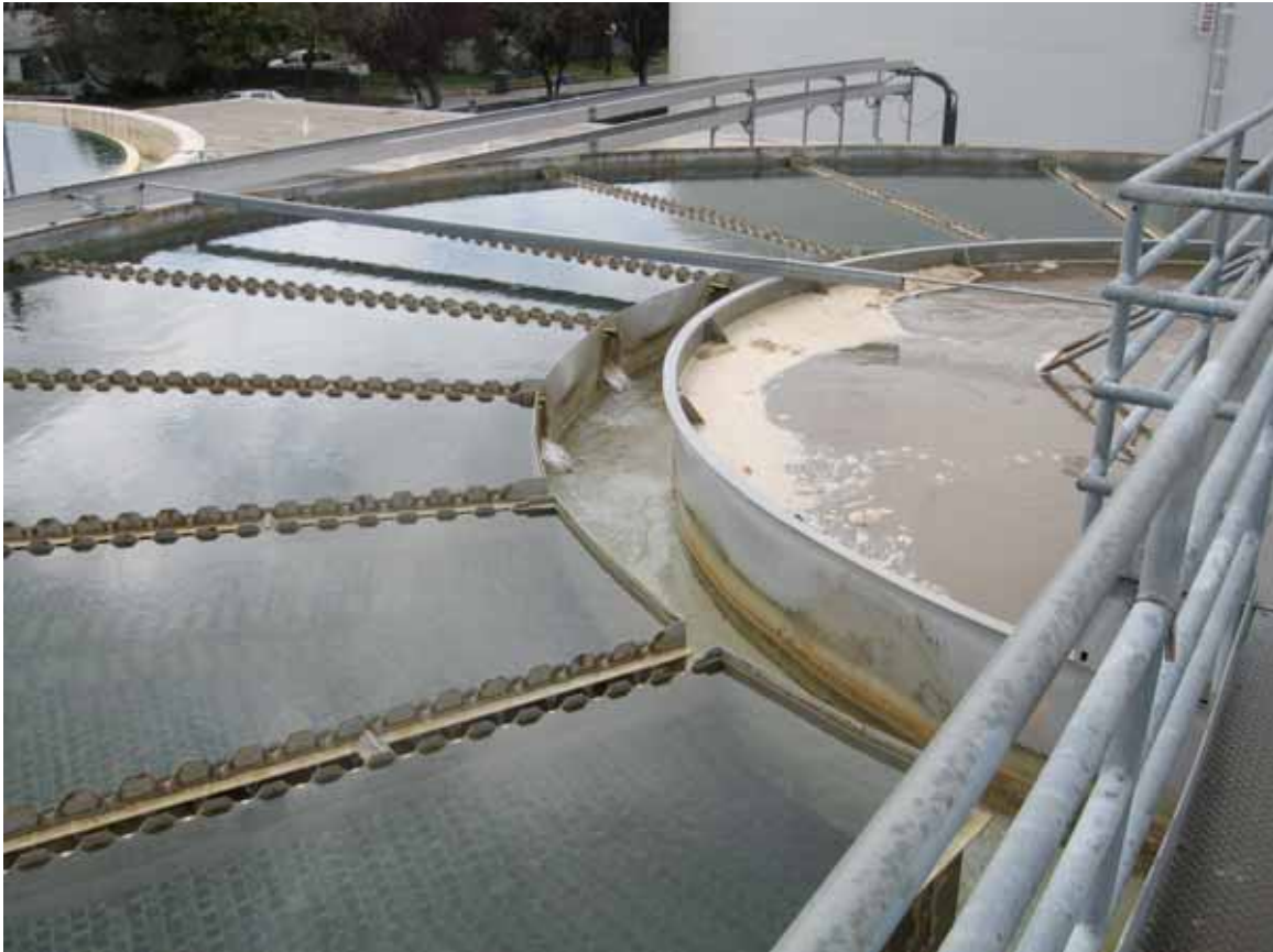
Figure 5-16. Accelerator 2 Tube Settlers and Launders
