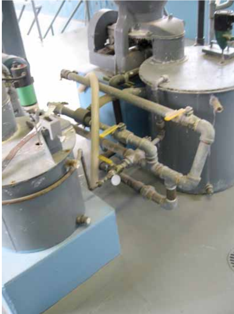
Figure 5-12. Unrestrained Tanks within Chemical Building
