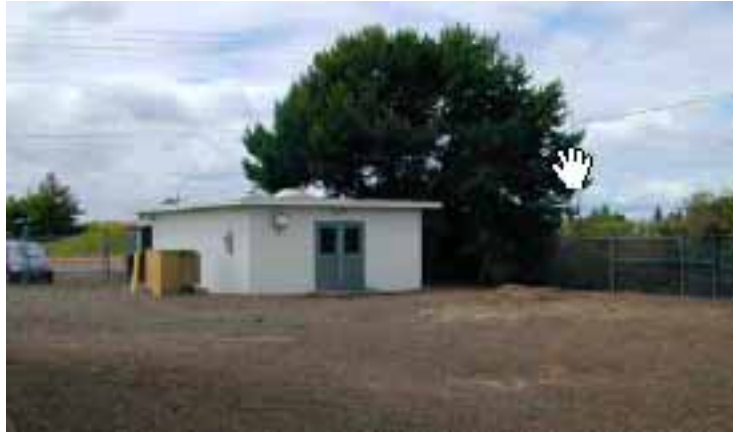
Figure 2-6. 34 th Avenue Pump Station
