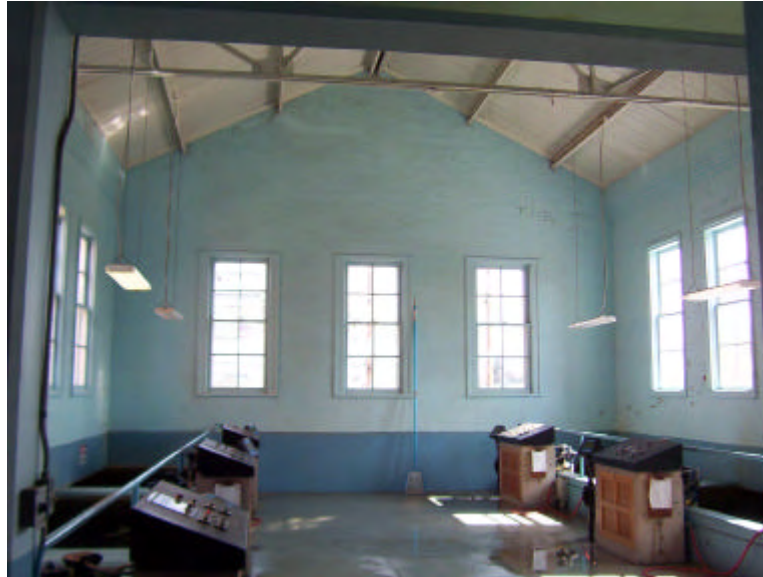
Figure 4.3-2: East wing interior looking east
