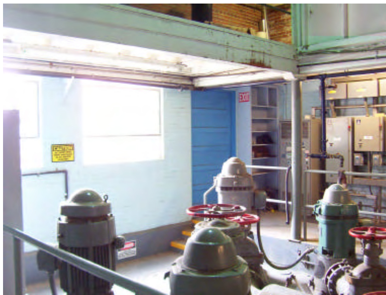
Figure 4.4-2: Interior looking southeast
