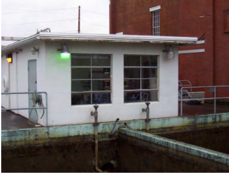
Figure 4.7-1: Large filter building, south elevation
