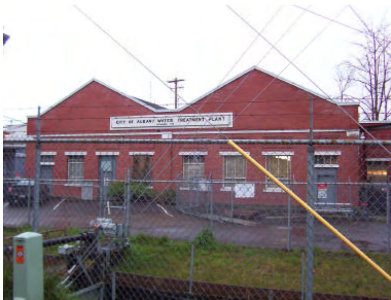
Figure 4.1-1: Control Building east elevation (entrance)
