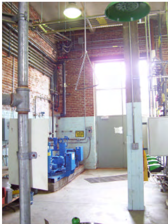
Figure 4.2 -2: Soda Ash first floor interior, looking west
