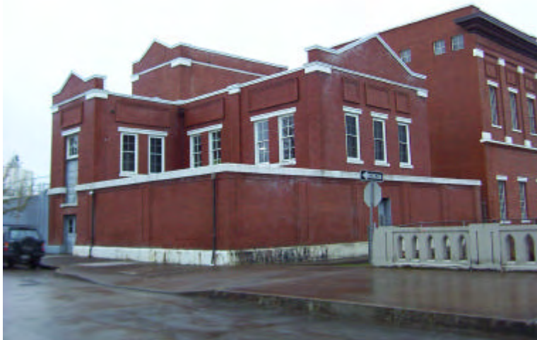
Figure 4.3-1: Old Filter Building looking northwest; note projection of central core above wings. Soda Ash building in background
