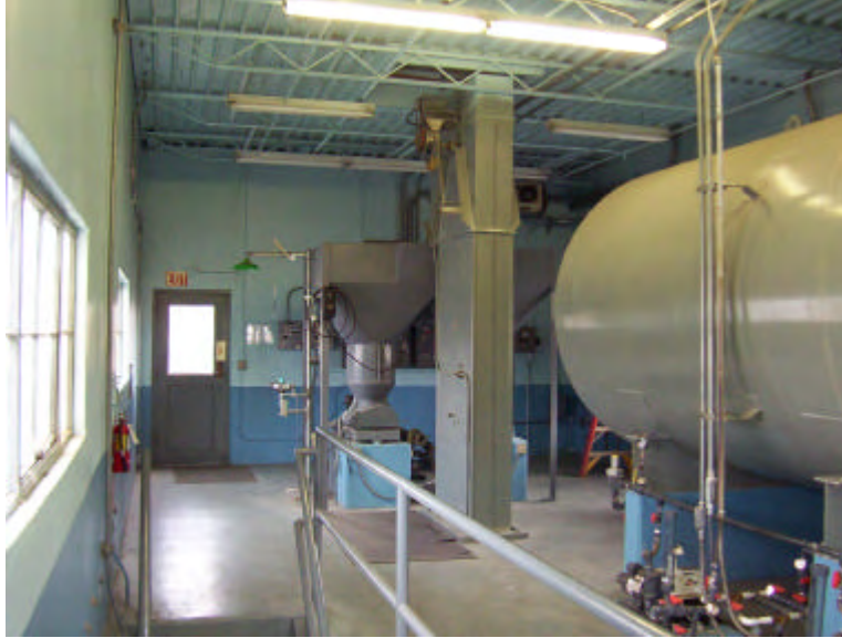
Figure 4.6-2: Interior second floor looking north
