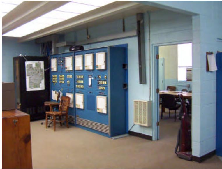
Figure 4.1-3: Interior of conditioned office space
