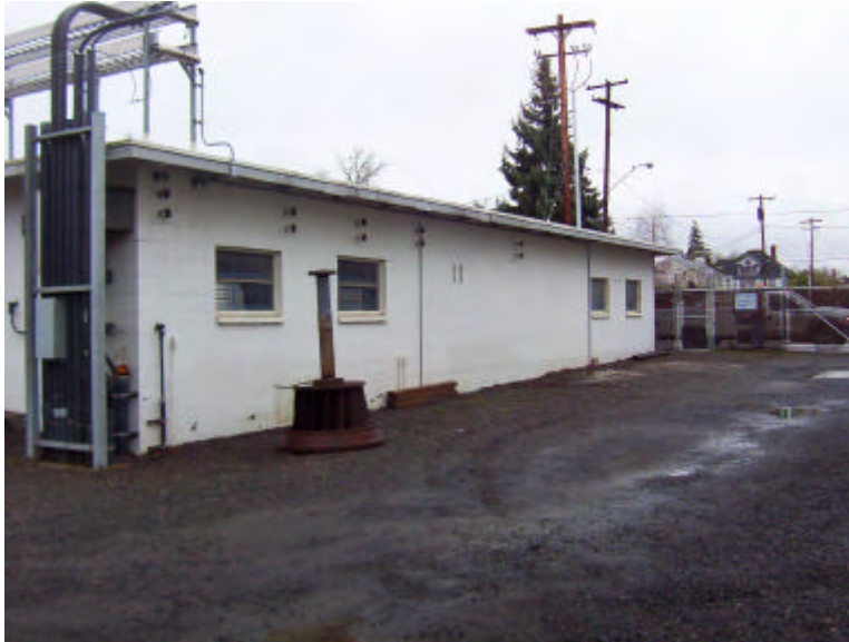
Figure 4.5-1: High Pressure Pumping Plant, west elevation
