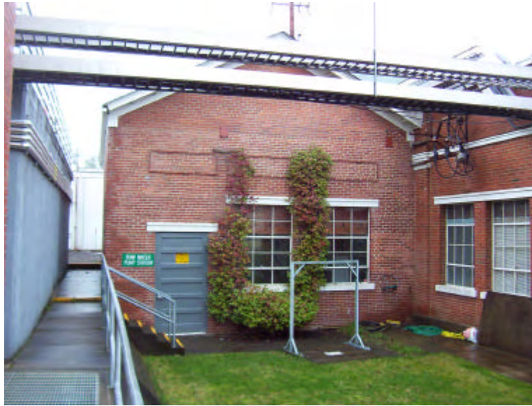
Figure 4.4-1: Raw Water Pumping Station building, east elevation
