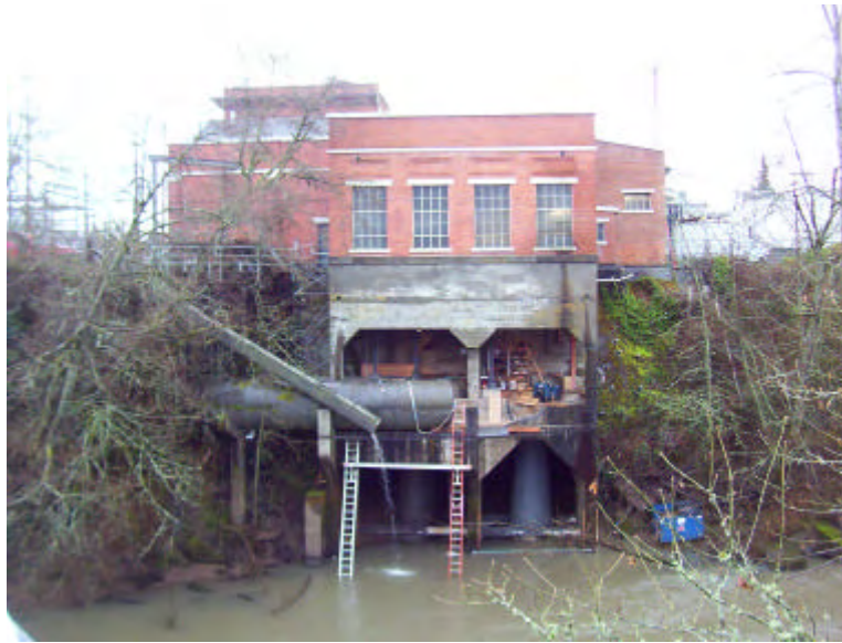
Figure 4.1-2: Control Building north elevation (north wing)
