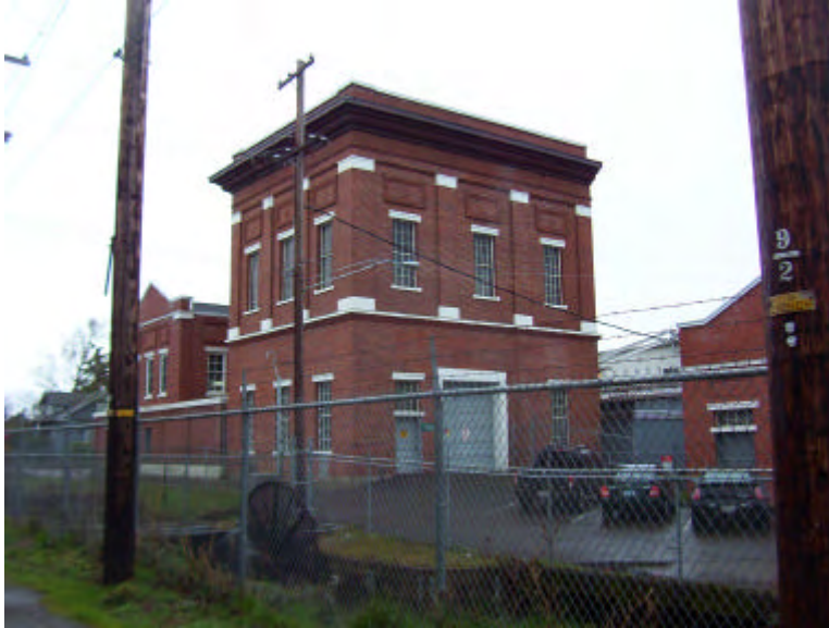
Figure 4.2 -1: Soda Ash building, north elevation
