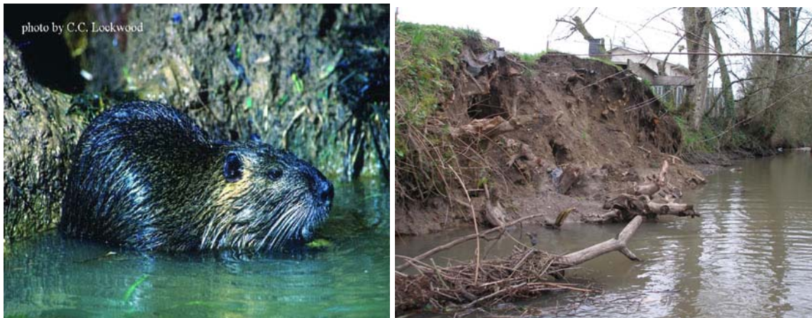
Figure 19: Nutria and Burrowing Damage Along Bank at Station 22+869
