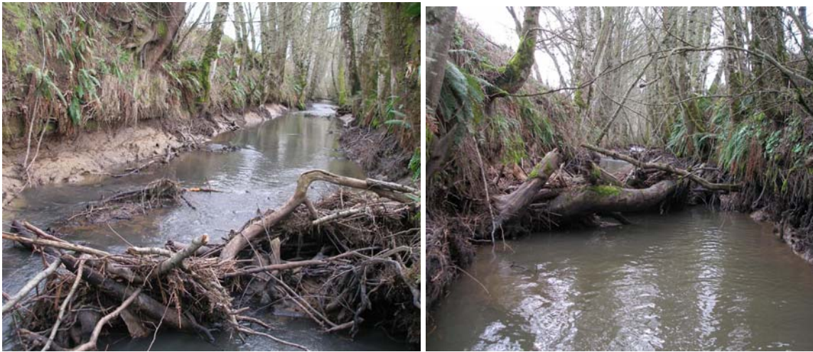
Figure 18: Debris Introduced Into Canal From Tree Failure Mechanisms
