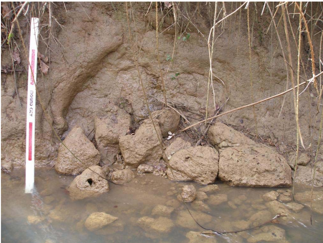
Figure 16: Disaggregation of Cohesive Bank Material from Freeze/Thaw Action
