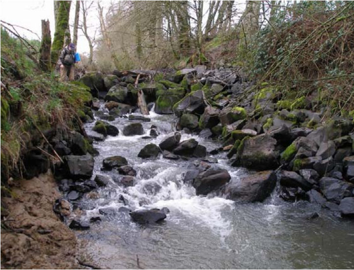
Figure 6: Grade Control Structure Upstream of Fry Road.
