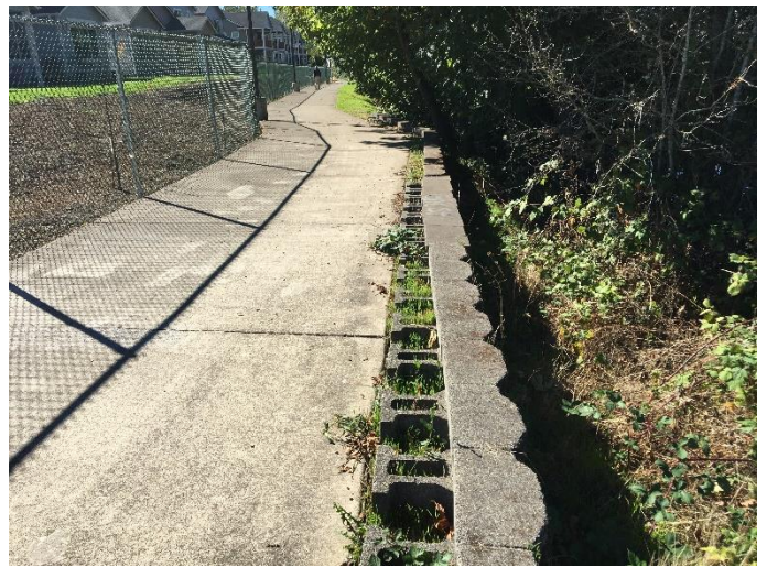
Between Madison & Hill, modular-block retaining wall, good trail condition
