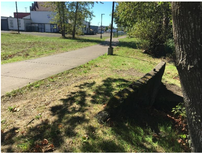
Between Thurston & Lafayette, good condition
