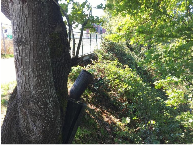
Between Jackson & Jefferson, tilting posts, pile-supported trail
