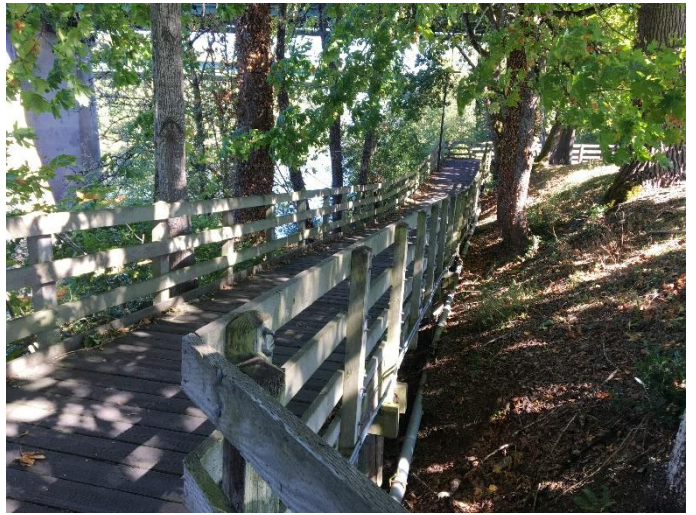
Between Broadalbin & Ellsworth, existing boardwalk
