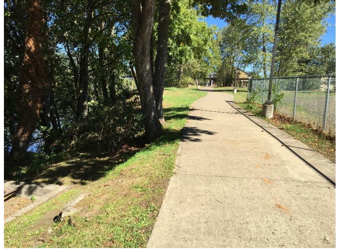
Between Jefferson & Thurston, good condition
