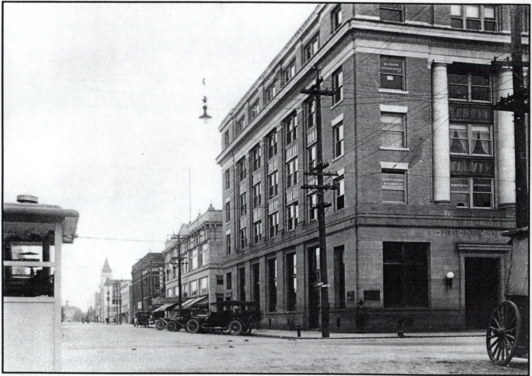
95) Albany's First National Bank Building on SW corner of First & Broadalbin. With upper stories removed it remains as First Interstate. Bank. Note popcorn stand at left, c. 1916.
