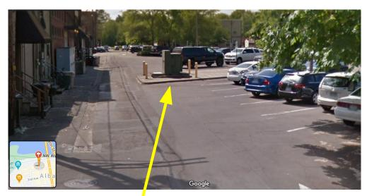
Pacific Power, 500 kVA Utility Transformer Adequate capacity is available per load review from the Utility Company.
