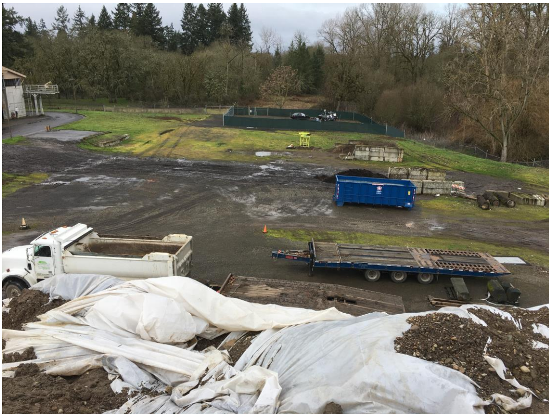
Photo 4A. Looking west from soil stockpile.
