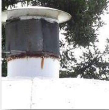
North Reservoir Vent 1
