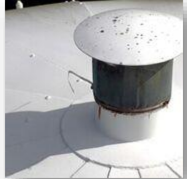
North Reservoir Vent 2
