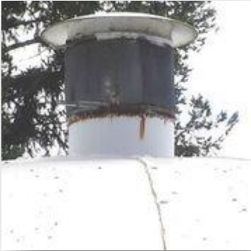
North Reservoir Vent 3
