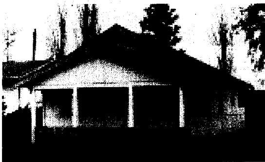
Unacceptable porch renovation #1- The porch floor has been removed, and the columns are supported by cinder blocks
