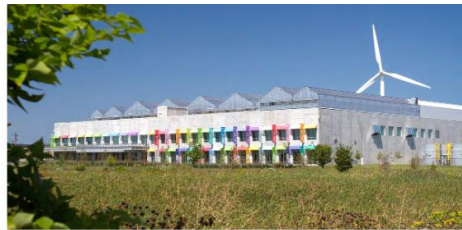
A 'green manufacturing' facility (sage production) with careful site planning, renewable energy and greenhouses on the roof
