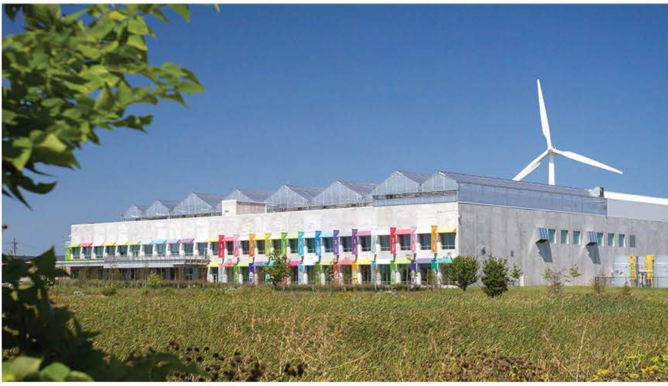
A "green manufacturing" facility (soap production) with careful site planning, renewable energy and greenhouses on the roof
