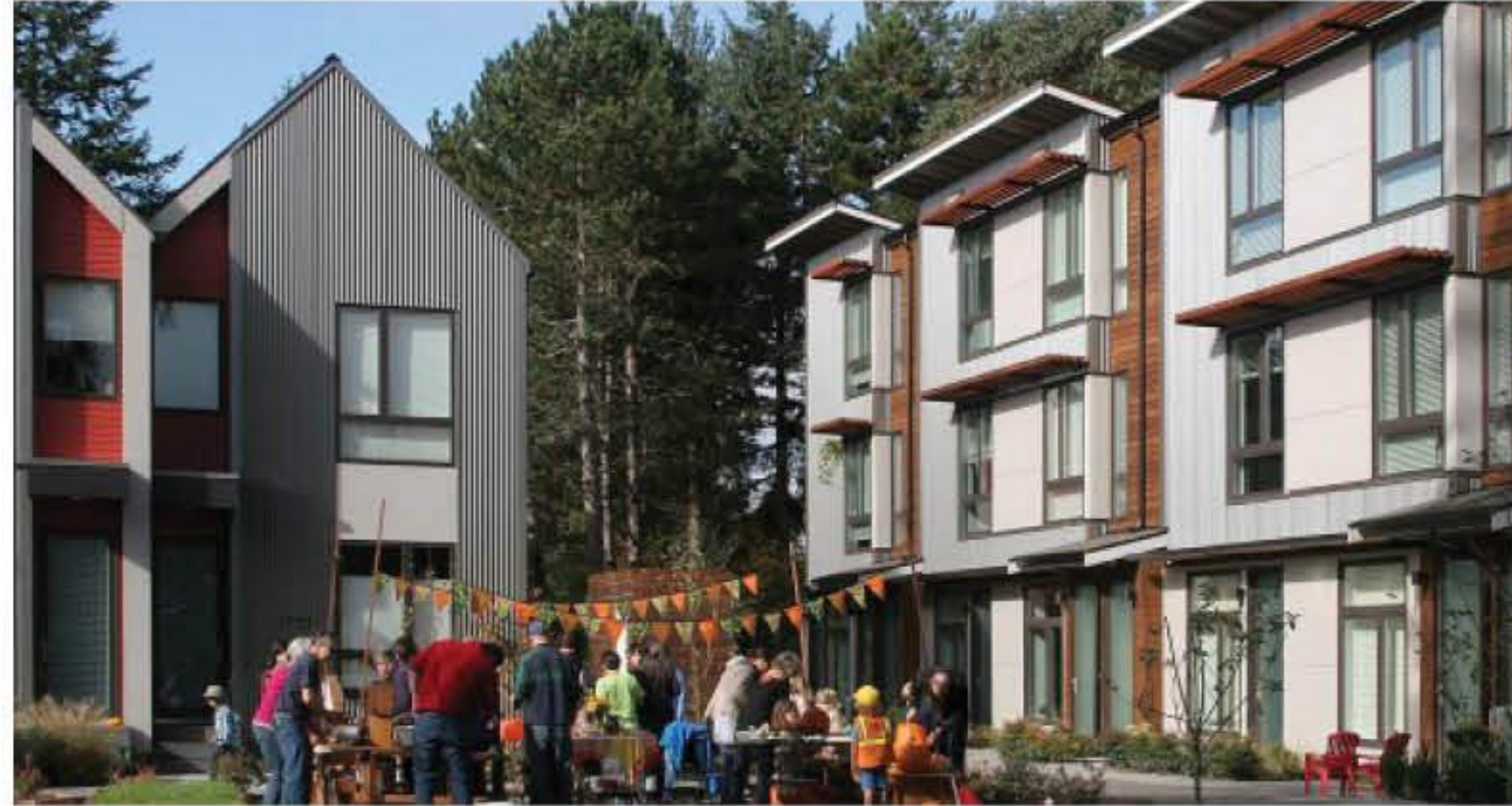
Example of high-density multi-family development, enclosing a courtyard with public gathering spaces.
