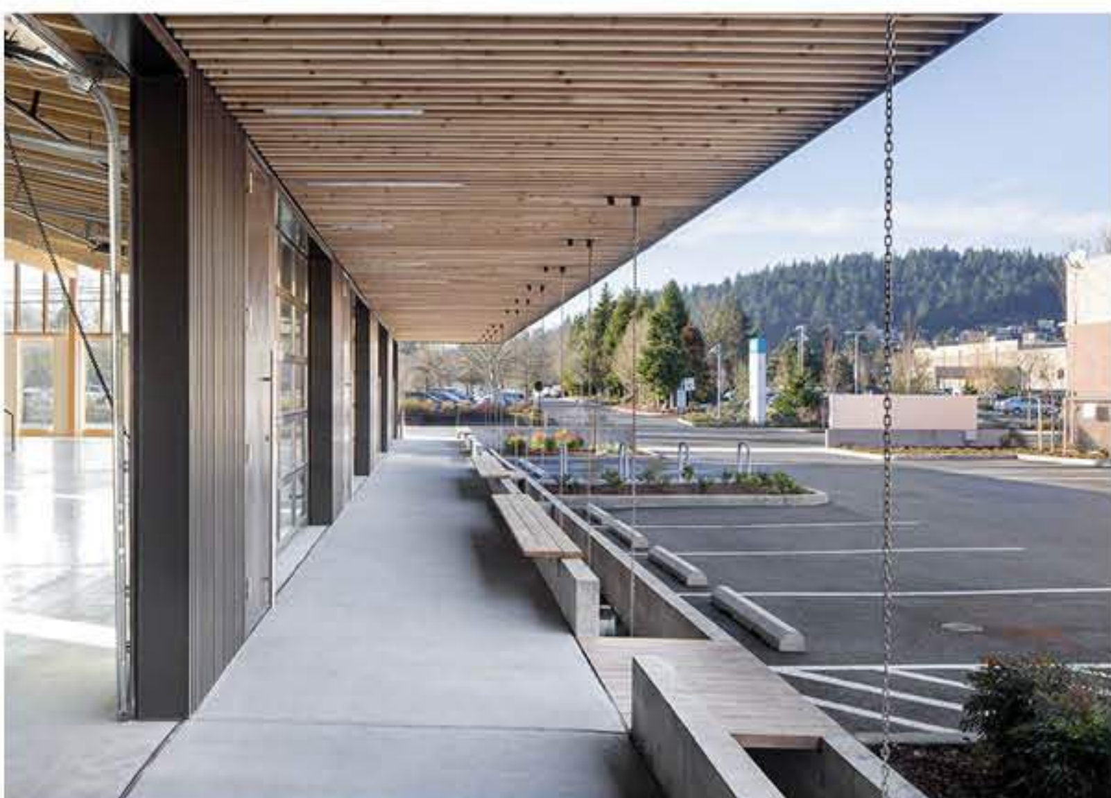
Flexible warehouse with stormwater planters and bike infrastructure integrated in parking areas
