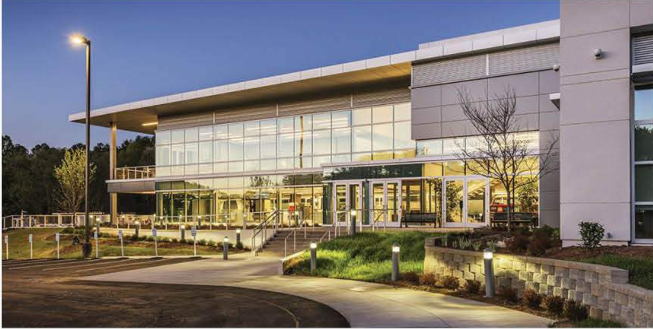
Multi-story office building with generous landscape and high-quality building design
