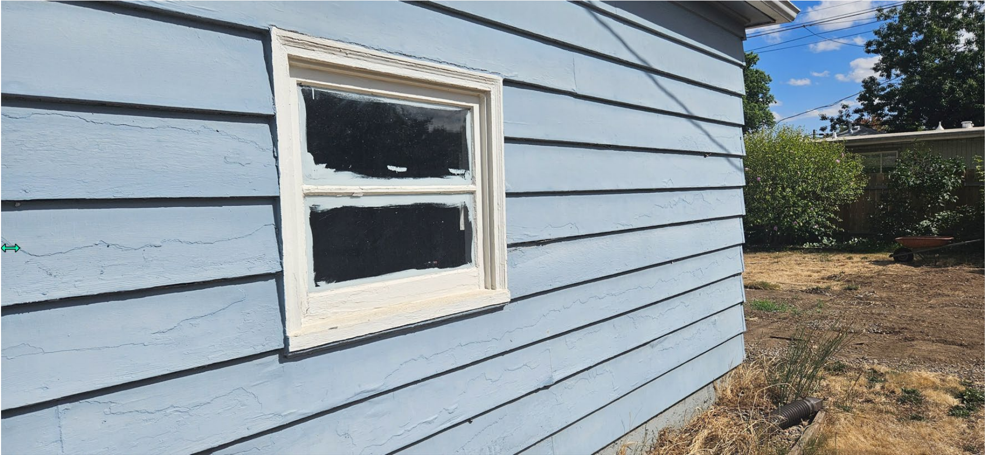
Figure 4: West Façade; Garage Window to be removed
