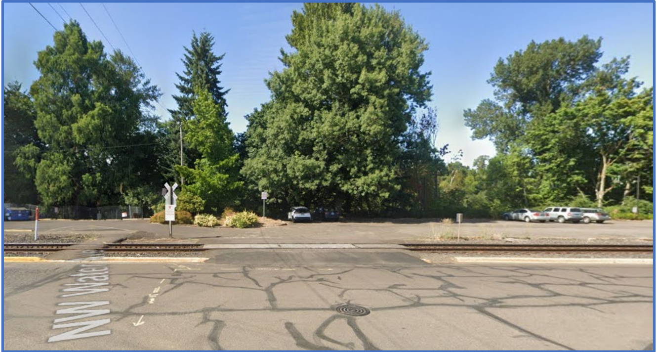
Figure 2b. At-Grade Rail Crossing at Intersection of Water Street & Ferry Street
