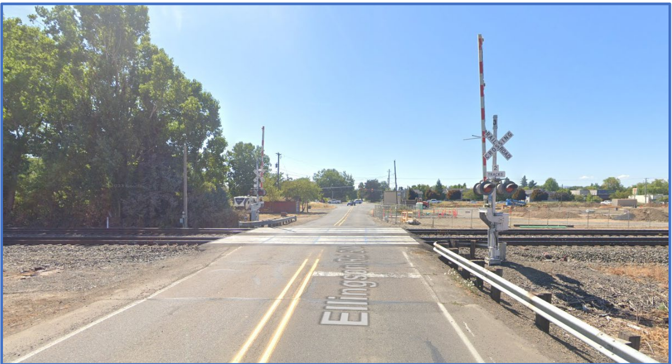
Figure 2. At-Grade Rail Crossing at Intersection of Ellingson Road, east of OR 99E
