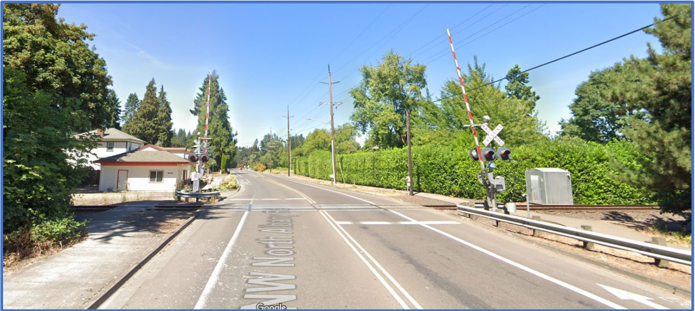
Figure 2. At-Grade Rail Crossing at North Albany Road
