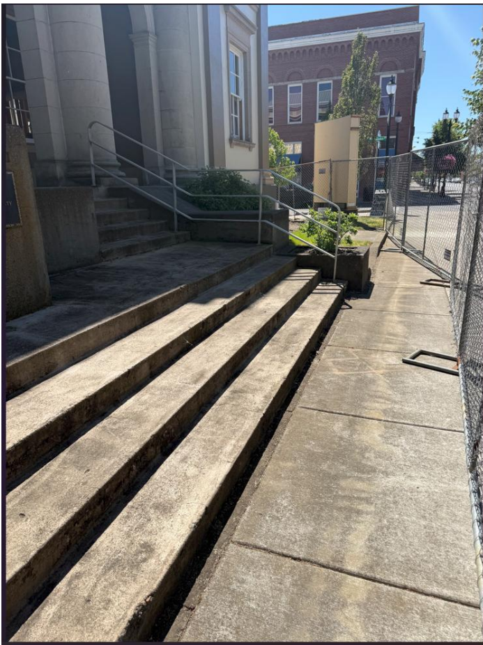
2 nd Avenue facing (north) entrance
