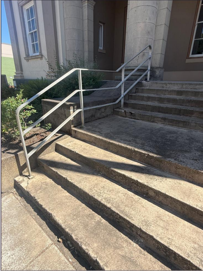
2 nd Avenue facing (north) entrance
