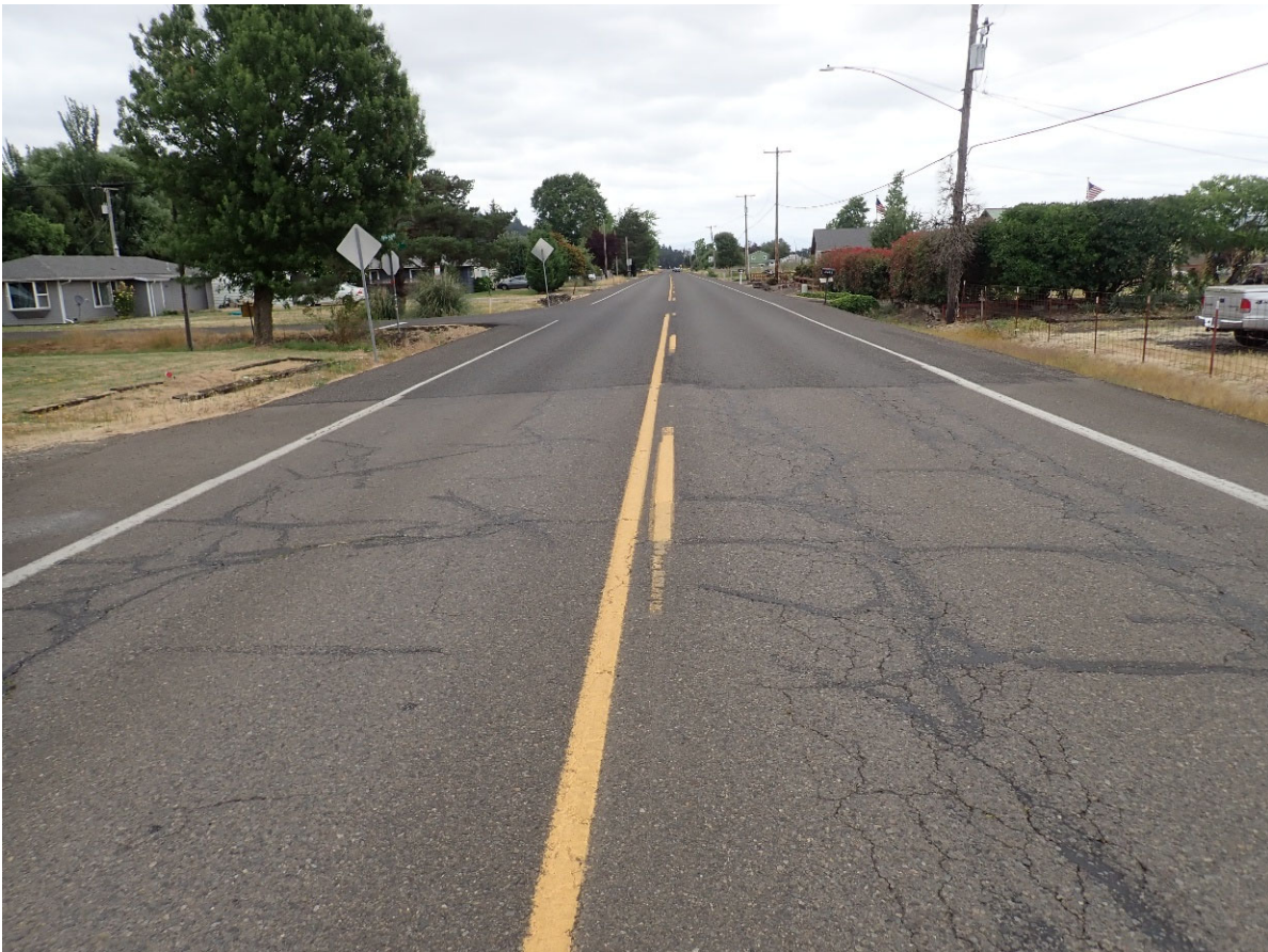
12. Looking eastbound from 100 feet west of Marilyn Street.
