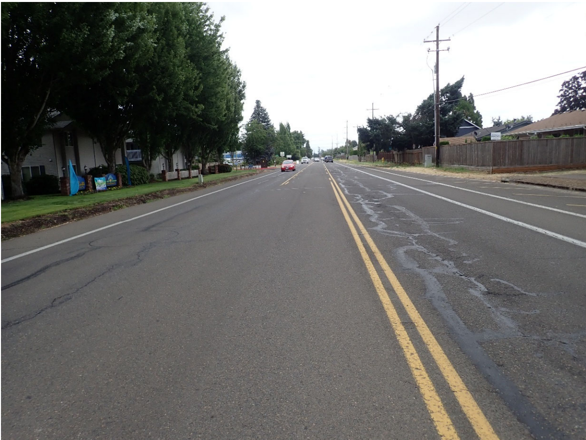
4. Looking eastbound from 200 feet east of Timber Street.
