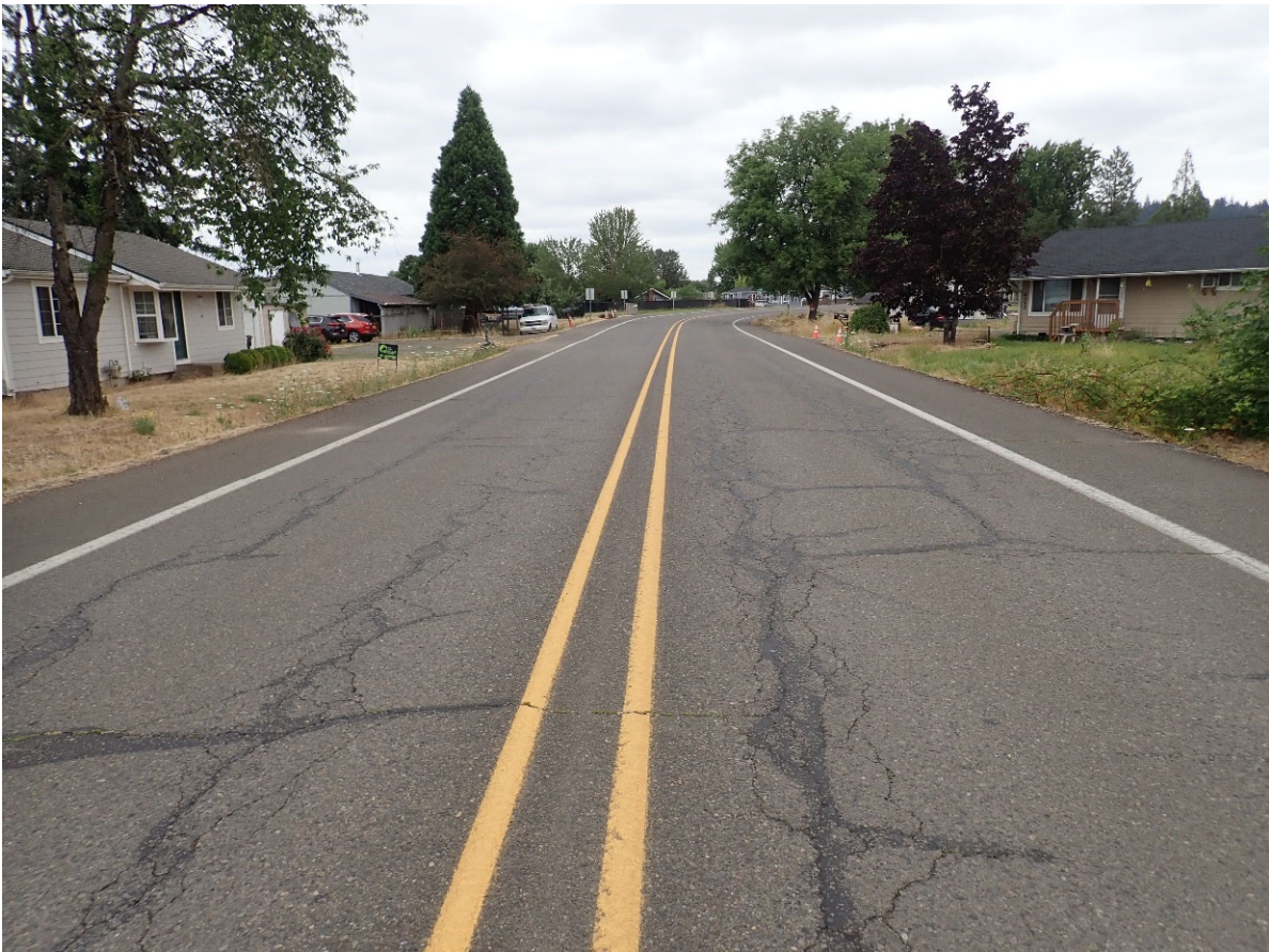
10. Looking eastbound from 300 feet east of San Felicia Avenue.
