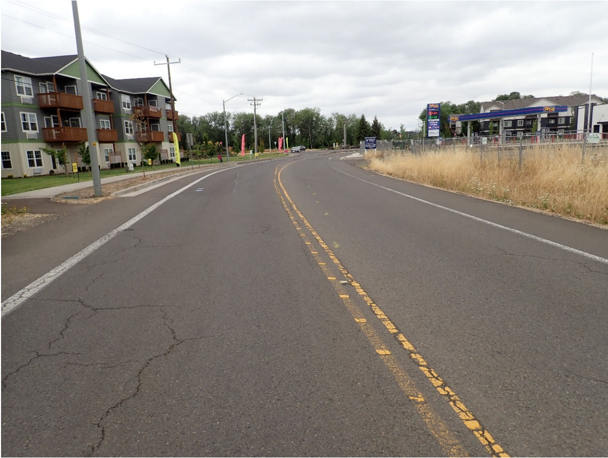
7. Looking westbound from 450 feet east of Timber Ridge Street.
