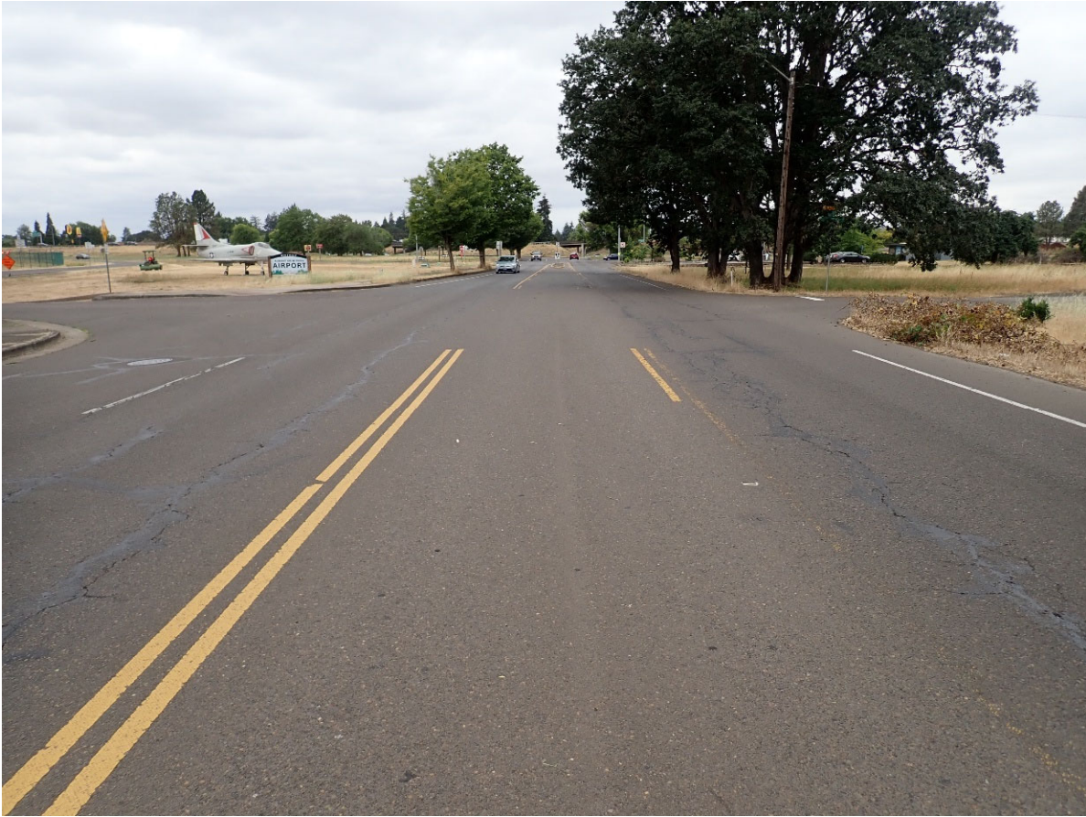
1. Looking westbound from 100 feet east of Aviation Way.
